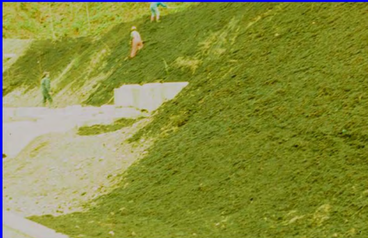
Compost blankets on steep slopes
